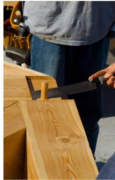
ABOVE: For a boathouse project in Cape May, NJ, that was designed in a collaboration between Hugh Lofting Timber Framing, the owner and an architect, pegs were trimmed in preparation for raising the bent, or end wall. BELOW: This custom carriage house, designed by Hugh Lofting, features three bays, a loft and a lower-level storage area. It is crafted of Douglas fir and finished with a pine tongue-and-groove ceiling, pine board-and-batten siding and hardwood flooring.
