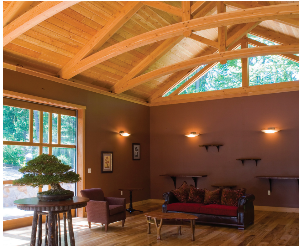
This structure features Douglas fir solid king-post trusses with a glued-laminated bottom chord. The ceiling is Douglas fir tongue-and-groove decking that provides a warm feeling and adds to the structural integrity.
