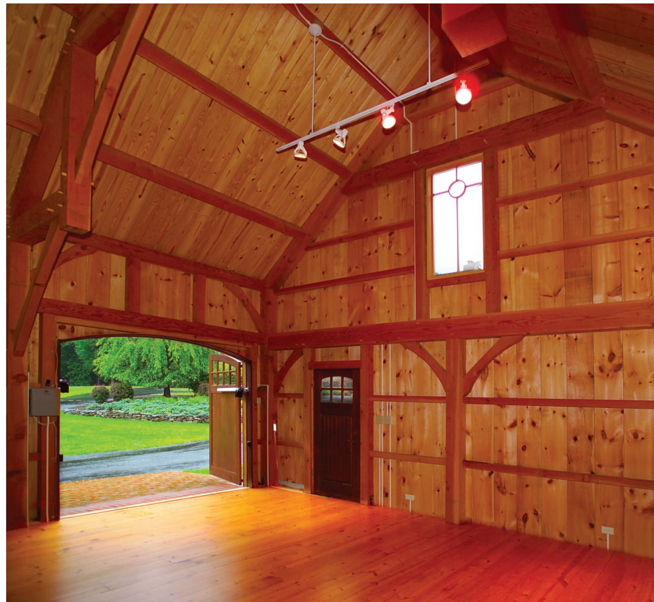
ABOVE: For a boathouse project in Cape May, NJ, that was designed in a collaboration between Hugh Lofting Timber Framing, the owner and an architect, pegs were trimmed in preparation for raising the bent, or end wall. BELOW: This custom carriage house, designed by Hugh Lofting, features three bays, a loft and a lower-level storage area. It is crafted of Douglas fir and finished with a pine tongue-and-groove ceiling, pine board-and-batten siding and hardwood flooring.
