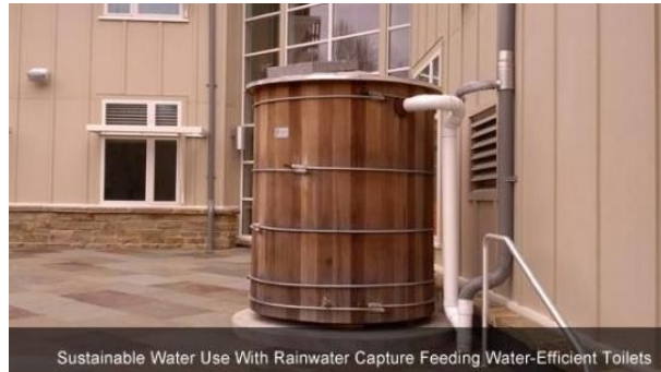
Sustainable Water Use With Rainwater Capture Feeding Water-Efficient Toilets
