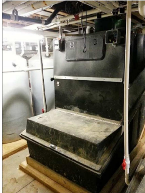
Clivus Multrum composter set below the toilets above in the bathrooms. There is a pair of these units in the mechanical room.
